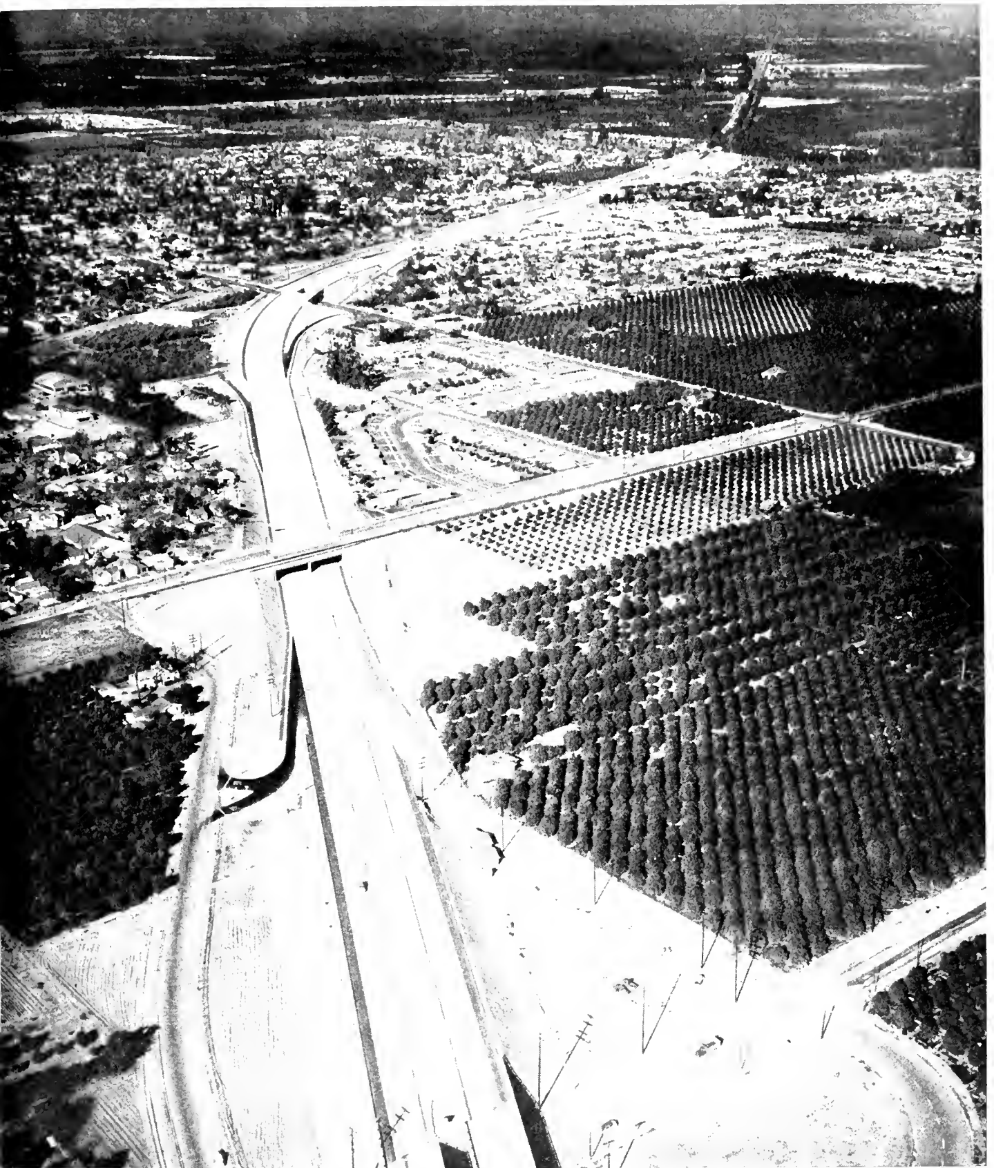
Looking northwesterly along Santa Ana Freeway, showing Grand Avenue Undercrossing in foreground, Lincoln Avenue Overcrossing and Santa Fe Railroad grade separation shown center left
